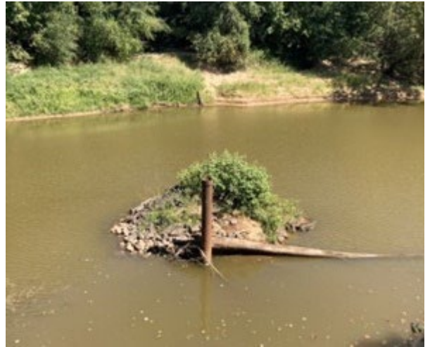
Figure 9: An orphaned well partially submerged in standing water.
