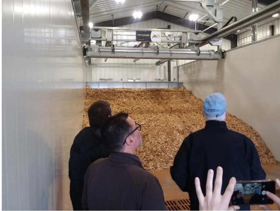
Wood chip storage for the Fond du Lac woody biomass district heating facility, commissioned in April 2018.
