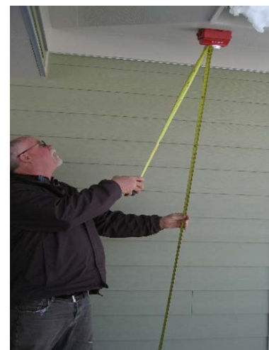
Facility Condition Assessment, Ute Mountain, Towaoc Colorado
