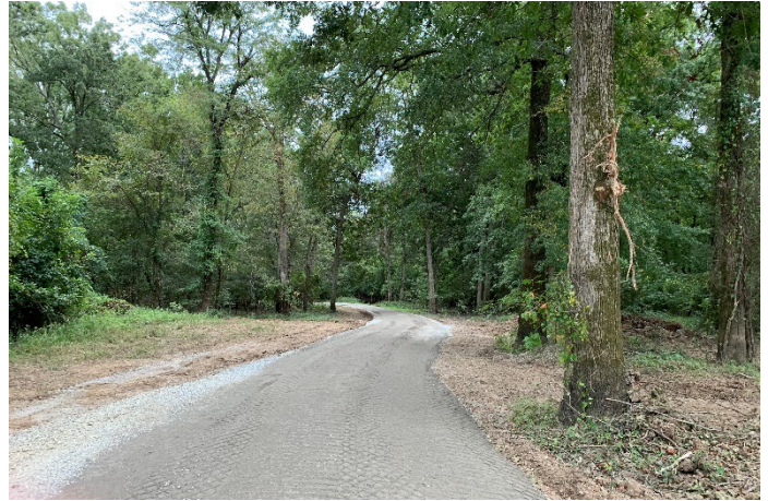
Figure 1. Dale Bumpers White River NWR – Passmore Road Rehabilitation
