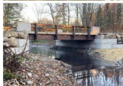
Perched culverts (top) are impassible by fish and other aquatic life. This newly constructed bridge (bottom) will allow aquatic life to reconnect with upstream habitats. Photo credit: USFWS
