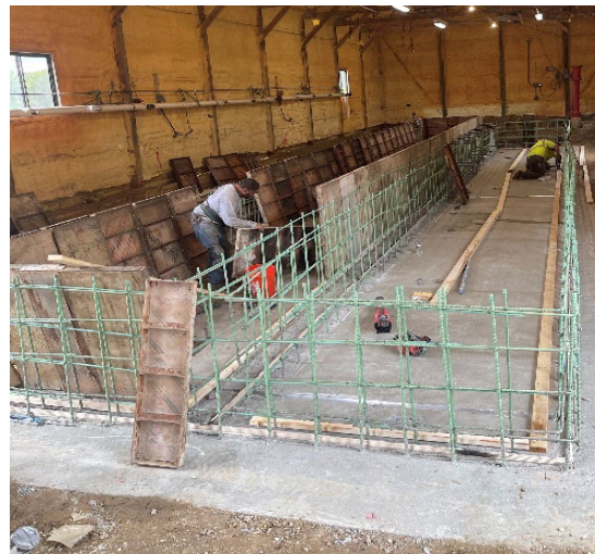
Genoa National Fish Hatchery, Wisconsin, replacing the old fiberglass indoor fish production raceways with long lasting concrete raceways. Photo credit: USFWS
