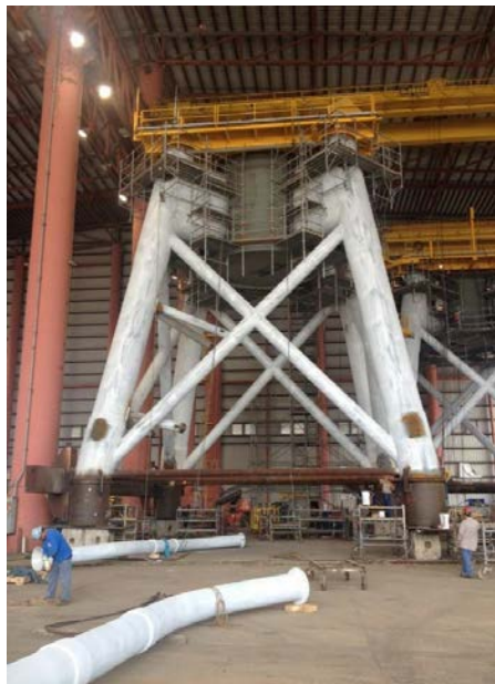
Fabrication of Block Island Foundations by Gulf Island Fabricators, in Houma, LA
