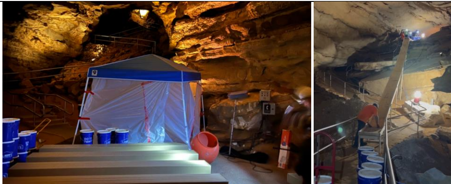
Workers staging construction materials inside Mammoth Cave.
