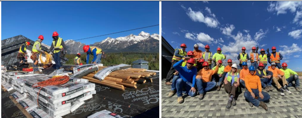
Left: Roof under construction. Right: Workers on completed roof.
