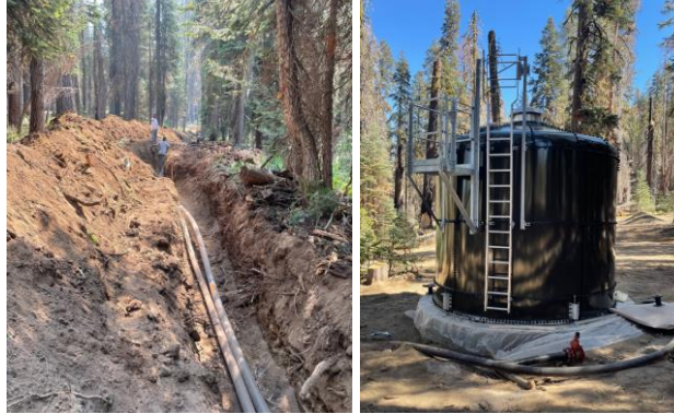
Left: Pipe installation in progress. Right: New water tank.
