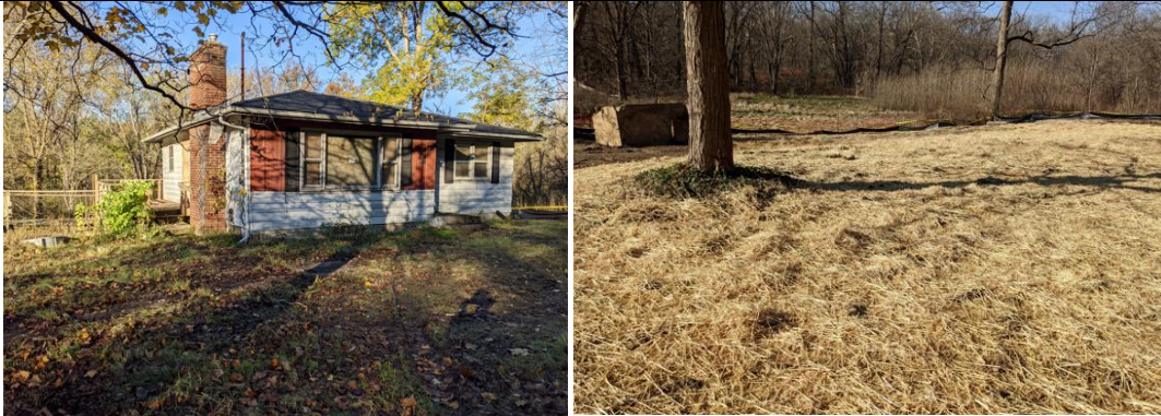
Left: Abandoned house. Right: Restored site after demolition.
