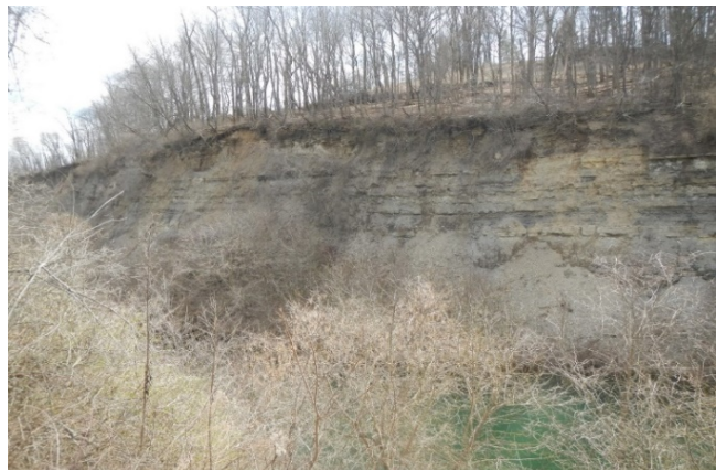
Deteriorating section of dangerous highwall just east of County Road 23 near Smithfield, Ohio
