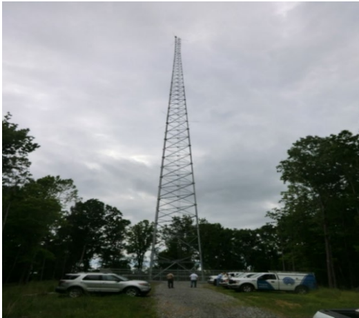
Broadband tower in place
