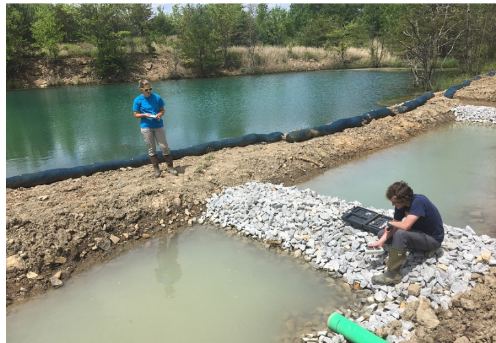
Beaver Creek Treatment Plant showing nearly complete settling ponds and wetland.
